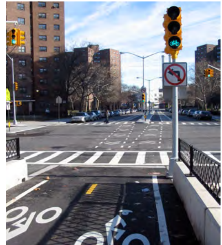
Figure 5-14: Example Median Path Striping
