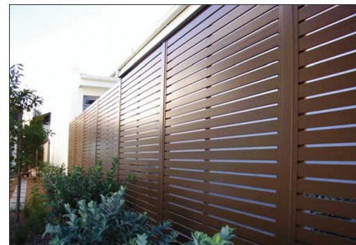
PRIVACY SCREEN SCALE: N.T.S. ALUMINUM W/ POLYMER WOOD PANEL FINISH
