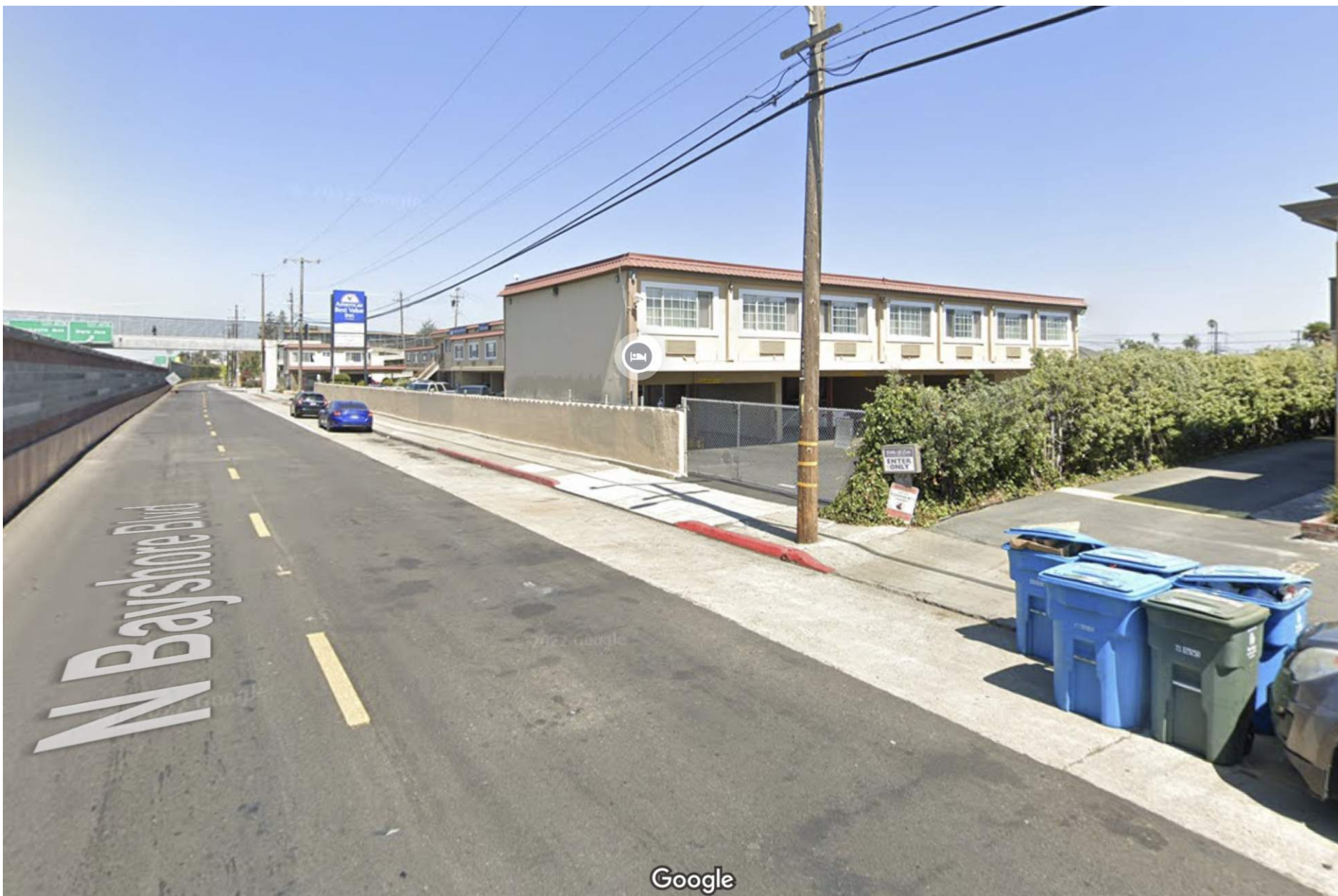
7. VIEW FROM N. BAYSHORE BLVD.
