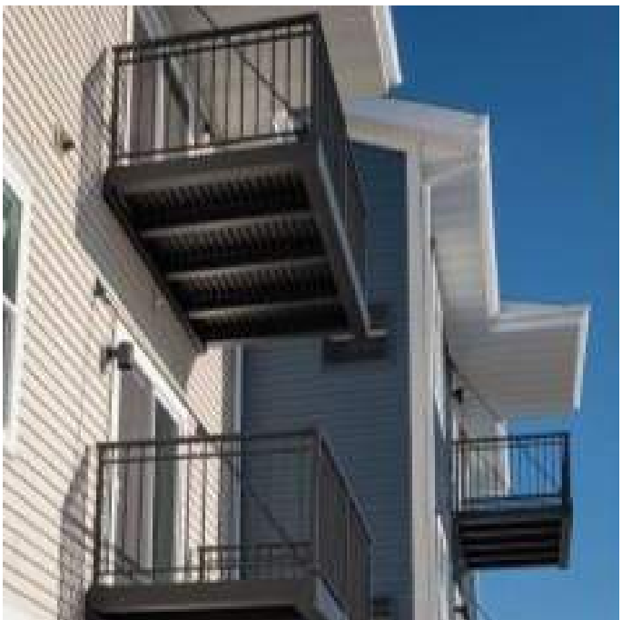
C-3 HUNG BALCONIES
