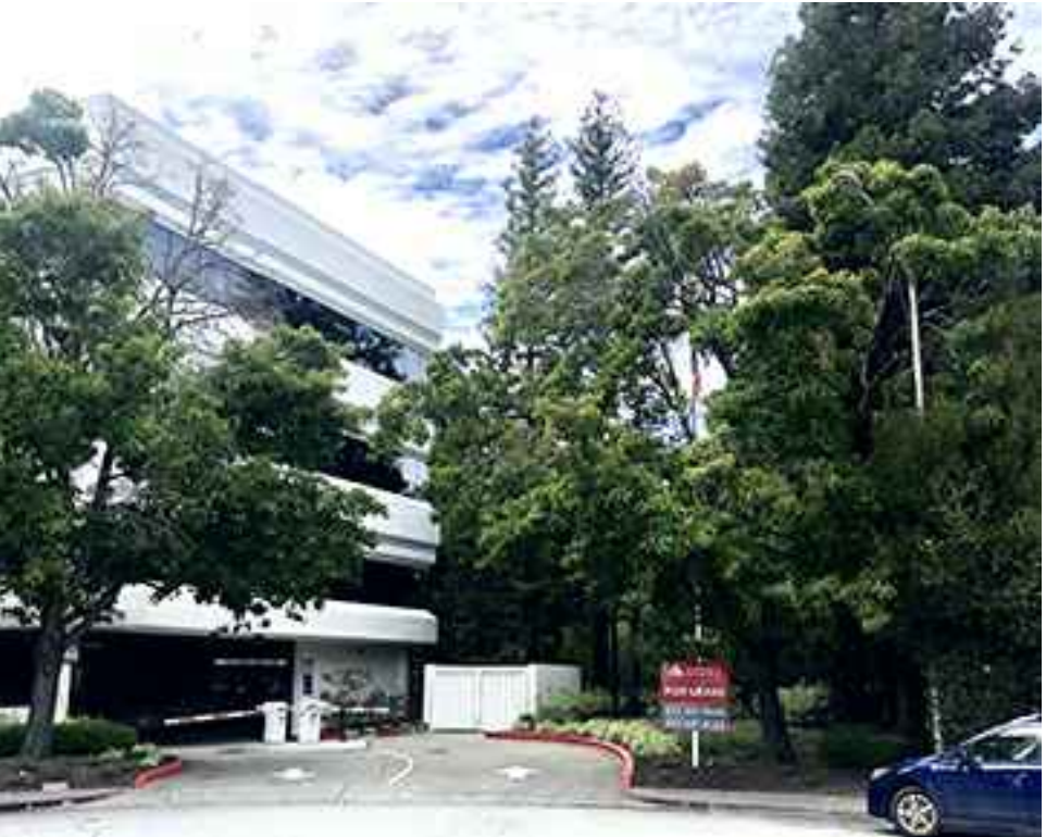
6 MID-RISE OFFICE DRIVEWAY
