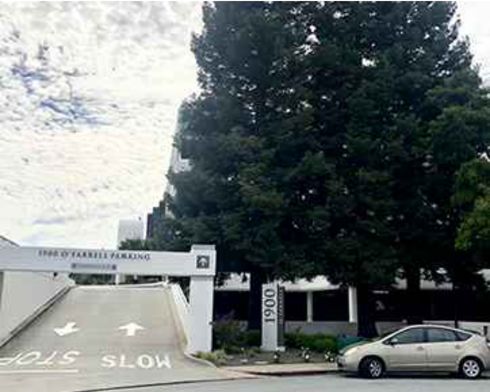
4 PARKING STRUCTURE SPEED RAMP
