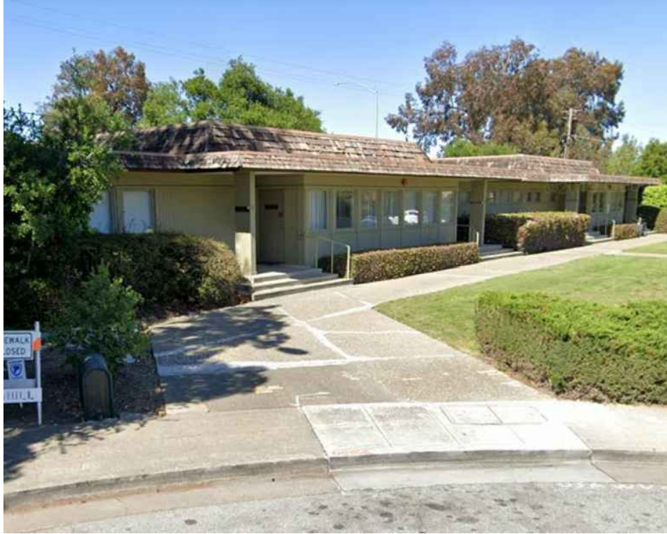
7 EXISTING SITE: BUILDING & WALKWAY
