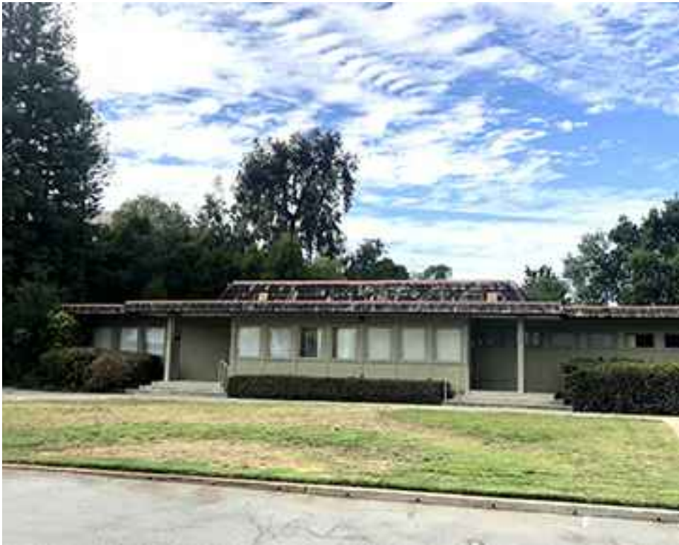
14 EXISTING SITE: BUILDING & LAWN
