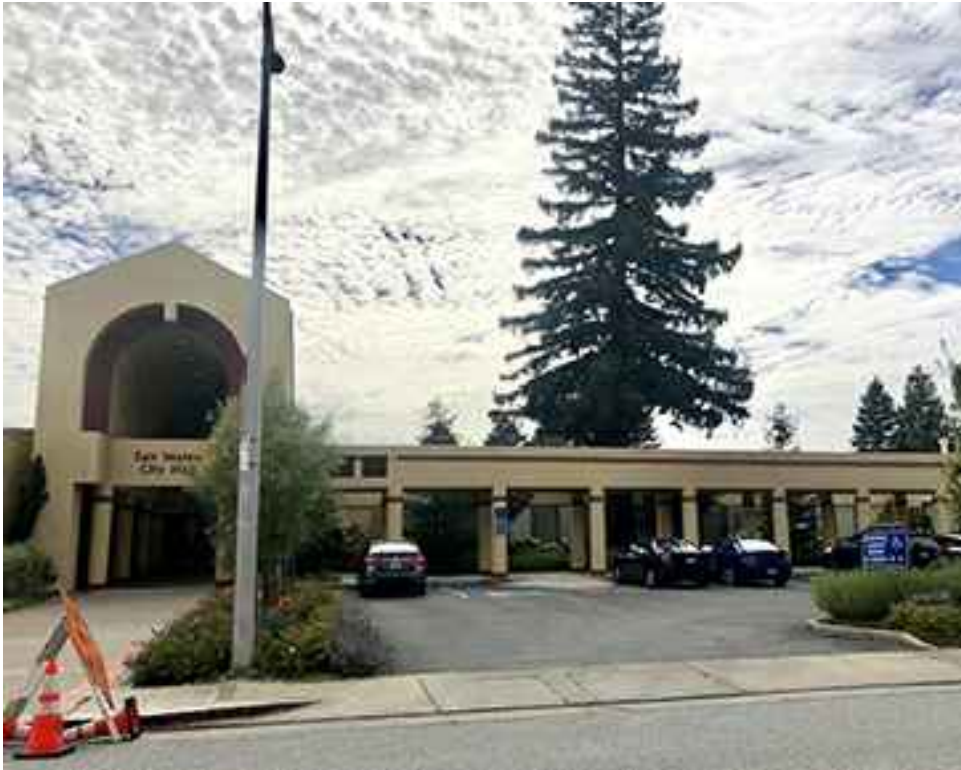
2 CITY HALL PARKING LOT
