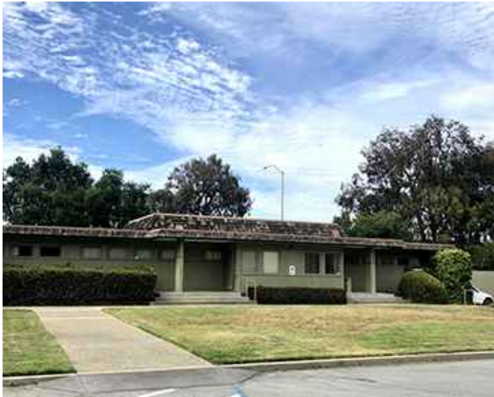
13 EXISTING SITE: BUILDING & LAWN
