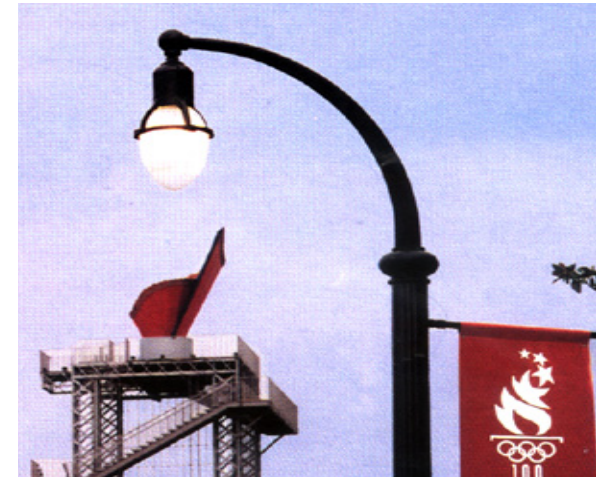
Figure 3.45 Close up of the Holophane Memphis Teardrop luminaire showing the option of an uplight and banner arm on the sidewalk (inboard) side of the pole.
