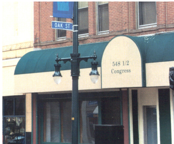
Figure 3.46 Holophane Pedestrian Teardrop Series lighting with two luminaires placed parallel to the street and a banner arm placed on the street (outboard) side of the pole.
