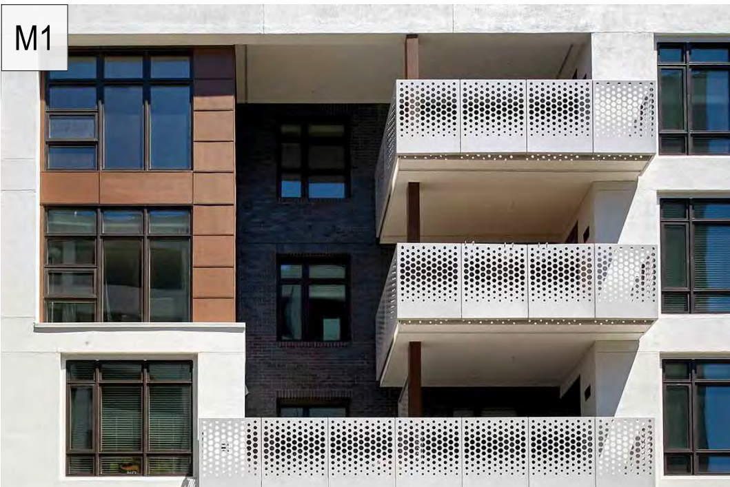
Metal Railing Example
