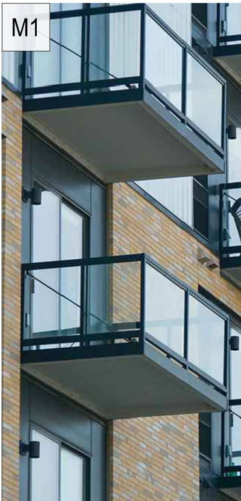
Metal Railing Example
