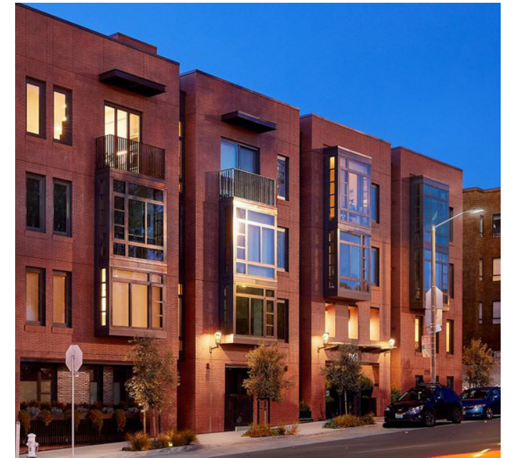
7.3.3 Figure 12 Vertical Wall Plane Break Example
