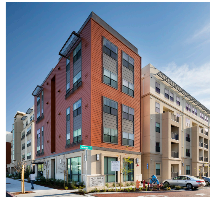
7.3.3 Figure 4 Stepped Parapets and Sunshades Example
