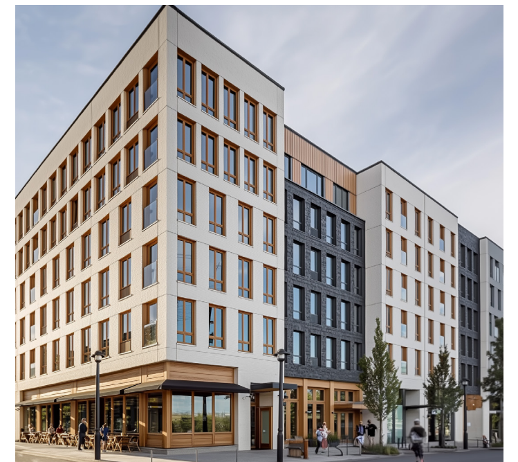
7.3.3 Figure 5 Glazing Pattern and Wall Plane Change Example
