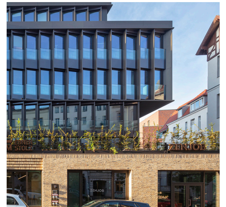
7.3.1 Figure 10 Stepback and Horizontal Reveal
