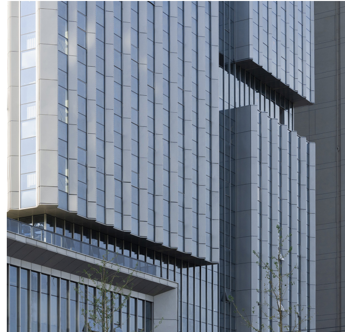
7.3.1 Figure 6 Vertical and Horizontal Reveals
