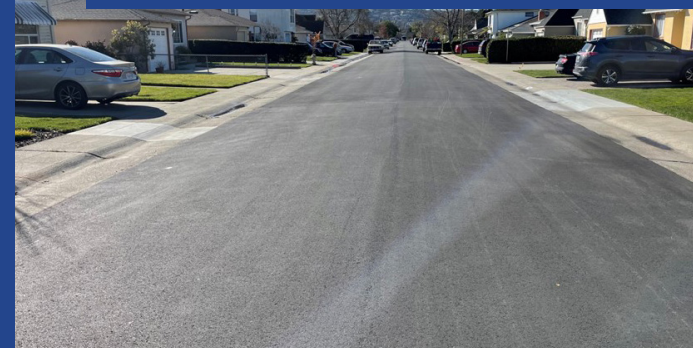
Figure 2: FDR with Asphalt Paving
