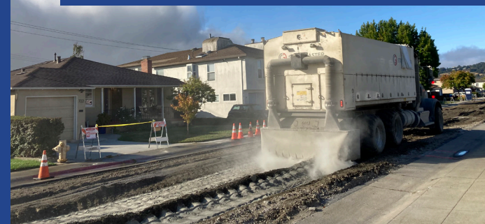
Figure 1: FDR Process During Construction
