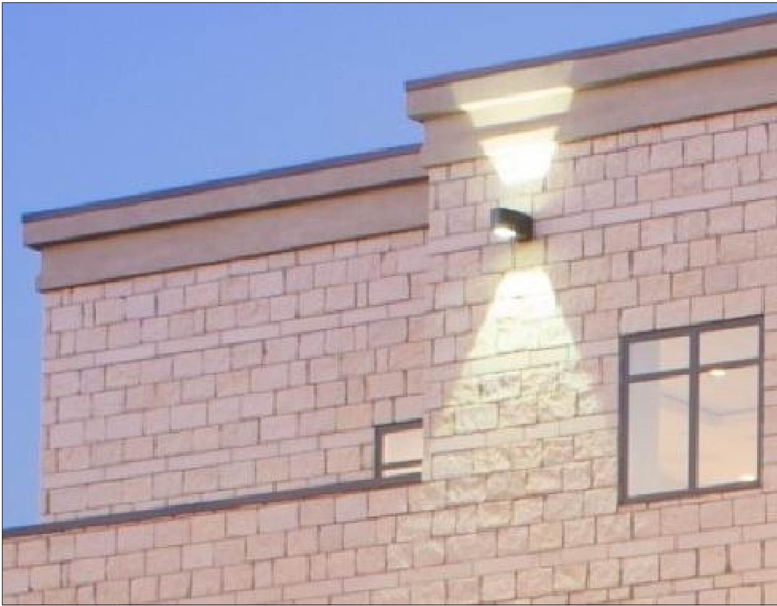
PRECAST STONE (SMOOTH EXT. SKIN O/ FOAM) CORNICE & BELLY BAND IN 'SIENNA'
