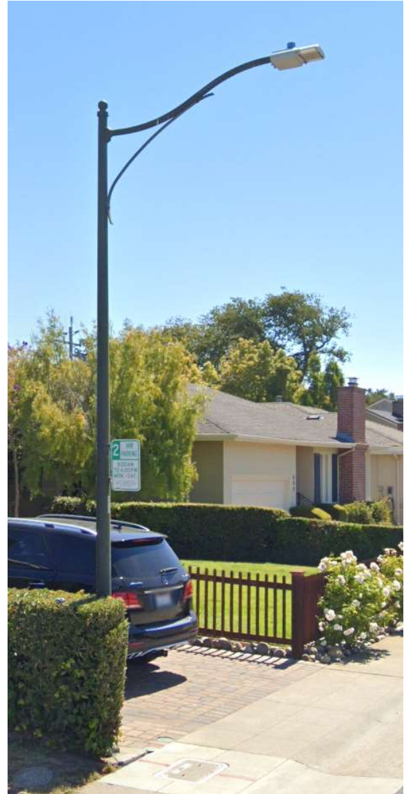
Green painted streetlight with LED cobrahead
