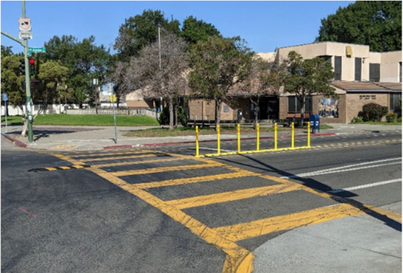
Figure 24: Centerline Hardening Example in Oakland, California
