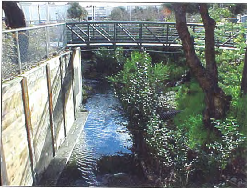
Photo 6-9: After emerging from the Edison Street culvert, the creek makes its way to El Camino Real in an engineered open channel alongside the Hillsdale Shopping Center.
