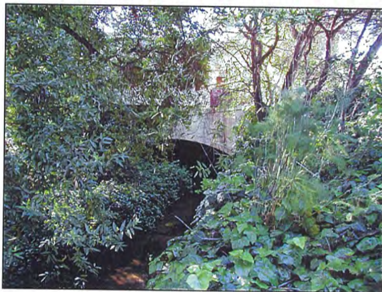
Photo 5-2: Entrance to San Mateo Creek Culvert at El Camino Real. Reservoir releases cause floodwater to leave the channel banks in this location.
