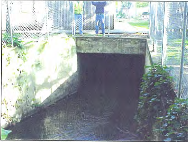
Photo 6-8: The natural creek disappears into an underground culvert beneath apartment buildings at Edison Street. Protecting the apartments and Hillsdale Shopping Center will require an additional underground culvert bypass.
