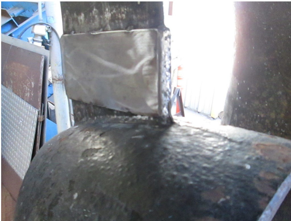
Pump suction bell stabilizer crack repair
