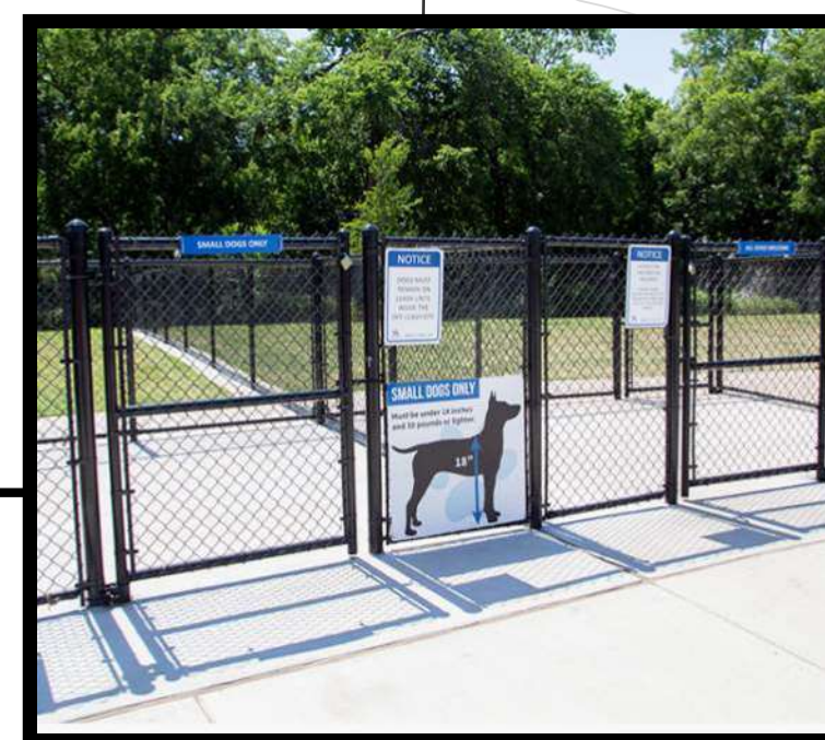
Dog Run Fencing - 5' H. Black Vinyl Coated Chain Link (2" Mesh) with Top and Bottom Rails
