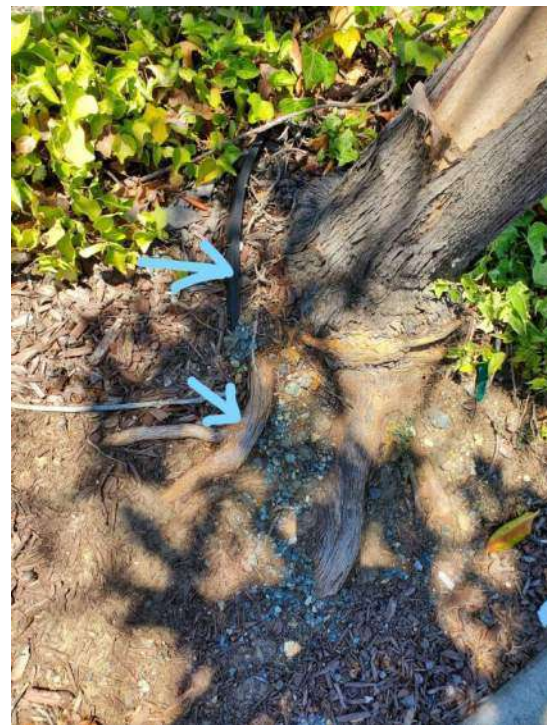
Root barrier and roots grown over barrier
