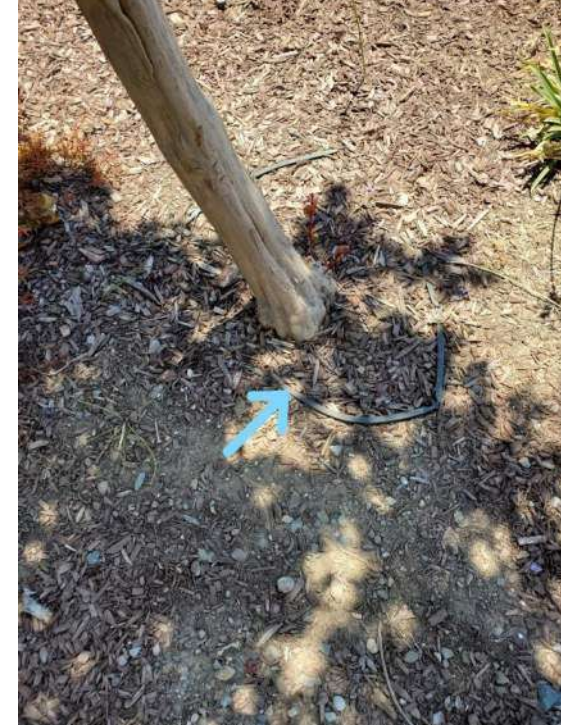
Root barrier and roots grown over barrier
