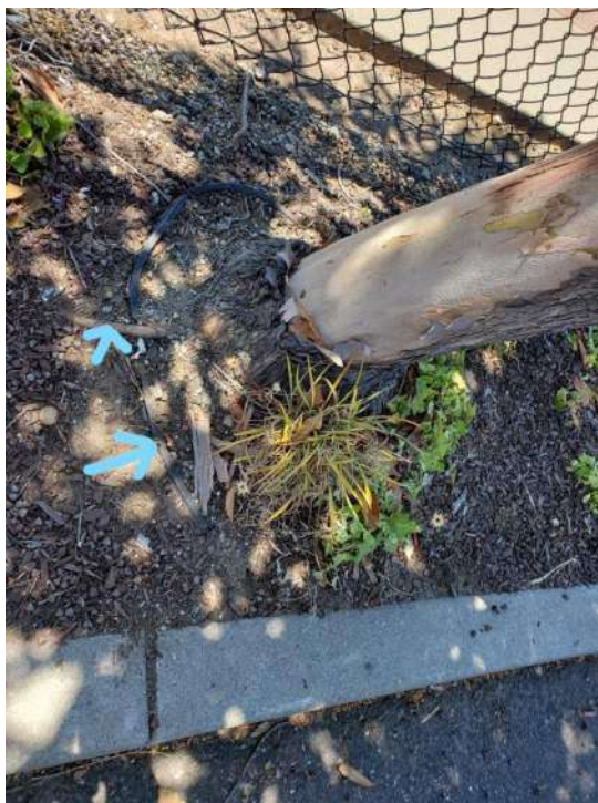
Root barrier and roots grown over barrier
