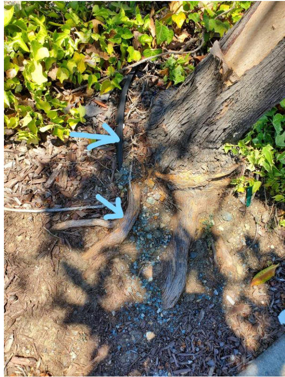
Root barrier and roots grown over barrier
