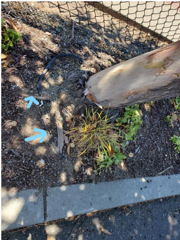
Root barrier and roots grown over barrier
