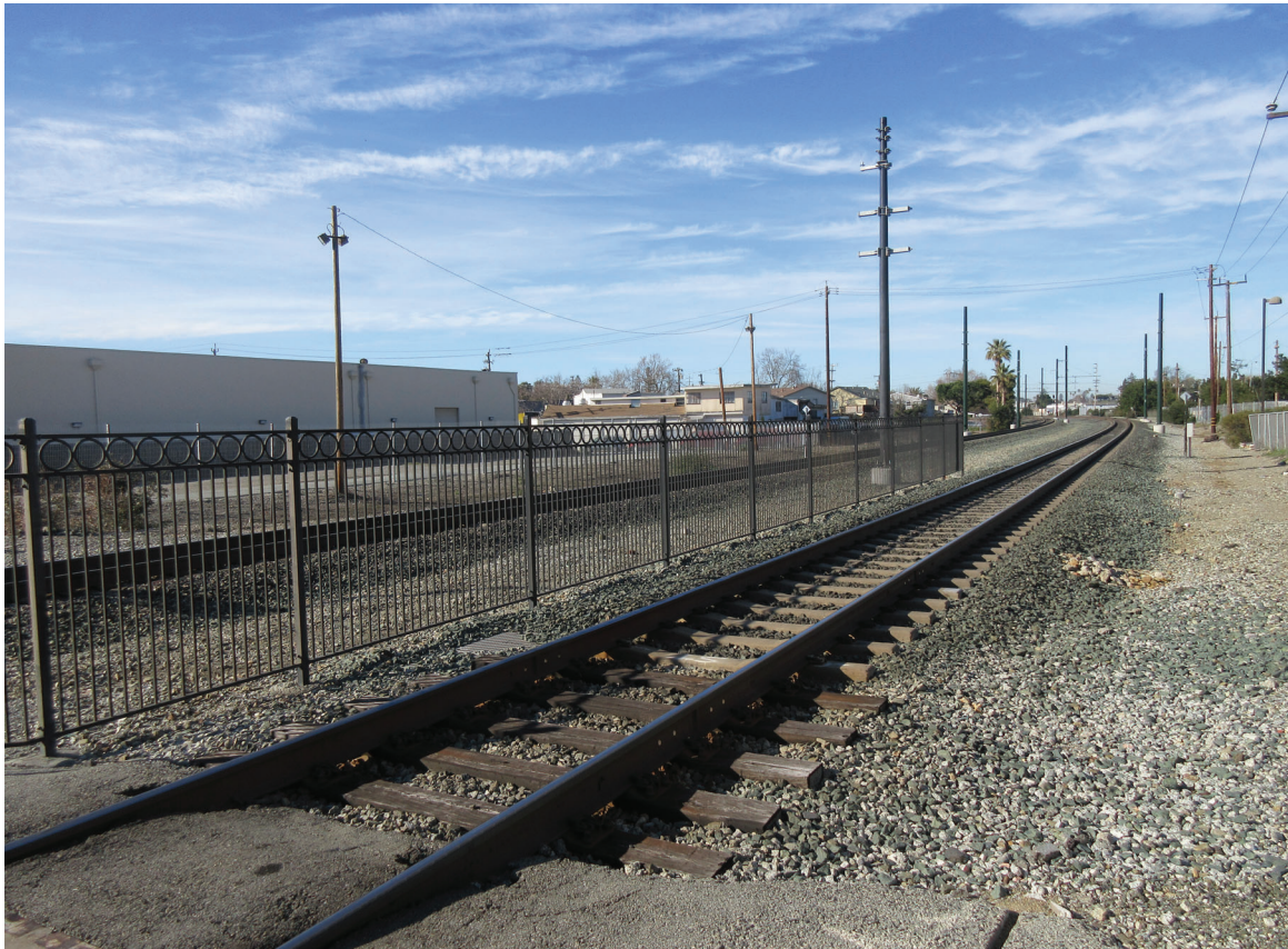
Photo 3: View of the railroad tracks looking north.
