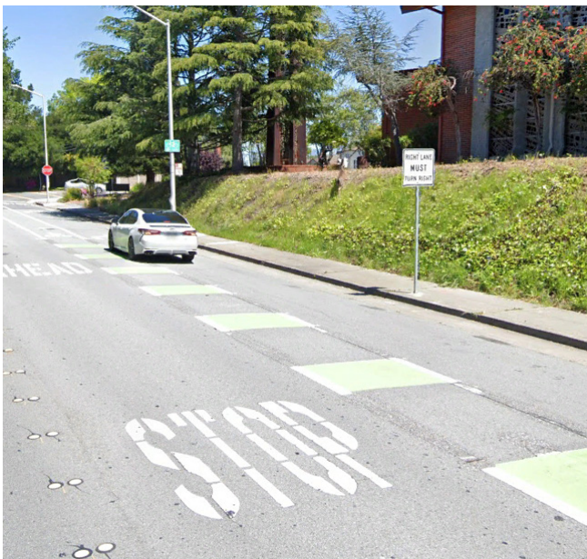
Figure 3.3: Painted conflict area markings on Crystal Springs Road
