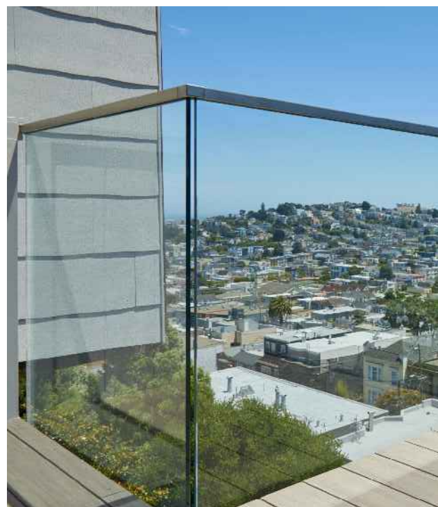
GLASS GUARDRAIL AT ROOF DECK
