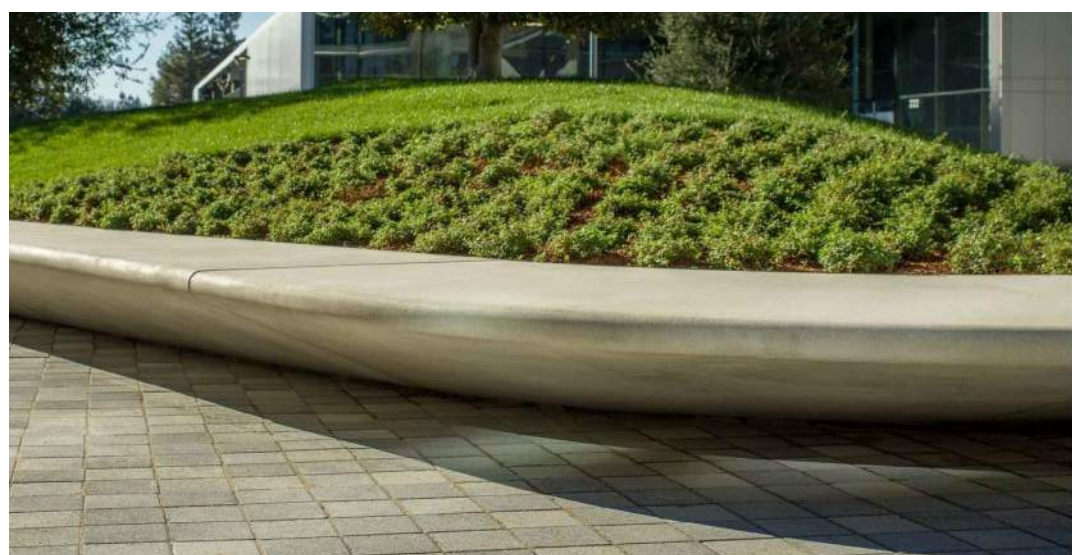
E4 Precast concrete planter and bench
