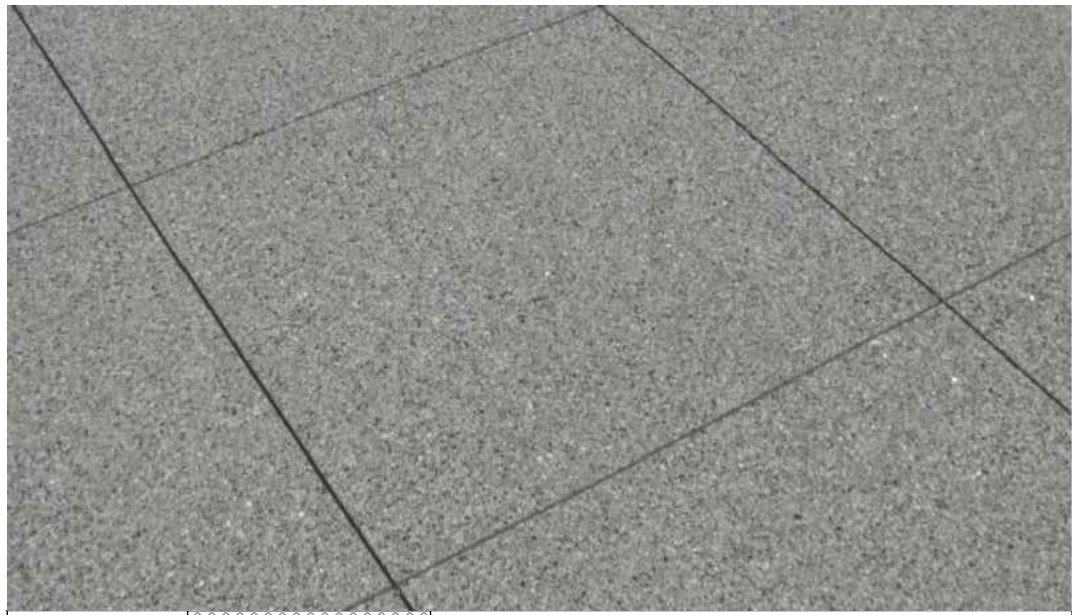
P2 CIP Concrete - Courtyard Paving
