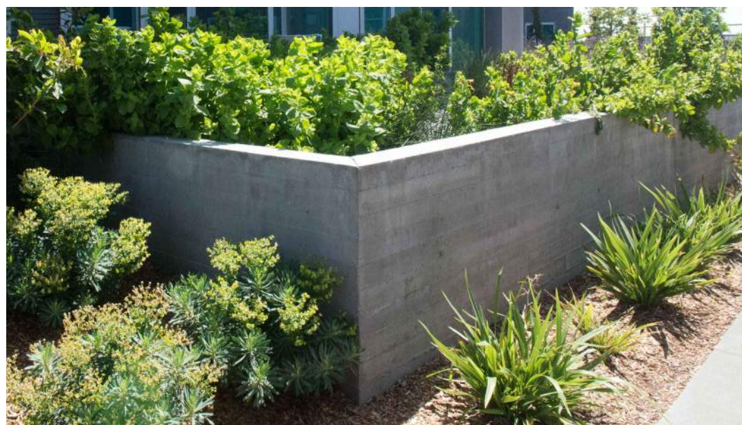
E2 Planter Wall B - Concrete at Residential Perimeter
