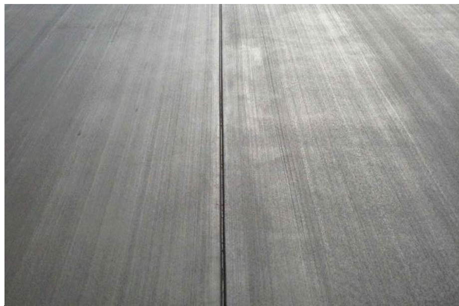
P3 CIP Concrete - Sidewalk & General
