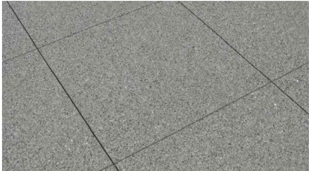
P2 CIP Concrete - Courtyard Paving
