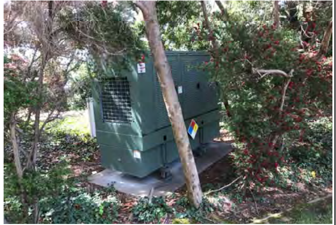
20. View of backup generator and associated diesel AST at the subject property, located south of POP 9.
