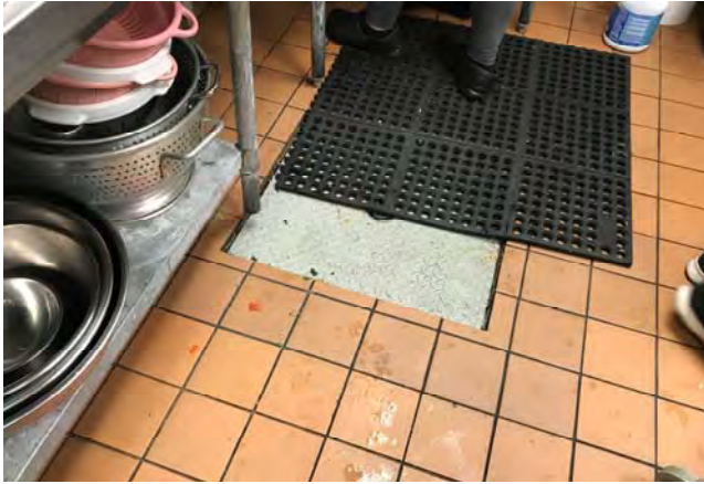
19. View of grease trap located in the kitchen of the café in POP 9.
