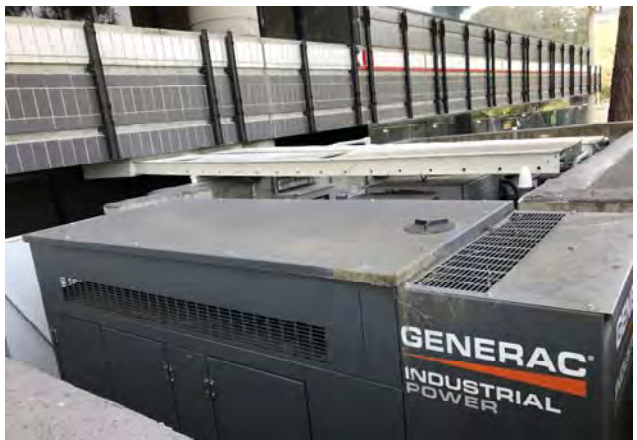
21. View of backup generator and associated diesel AST at the subject property, located at POP 8.
