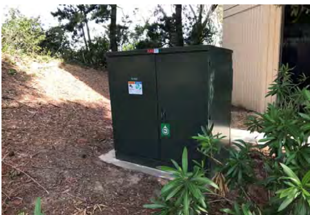
23. View of typical pad mounted transformer at the subject property.
