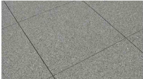
P2 CIP Concrete - Courtyard Paving
