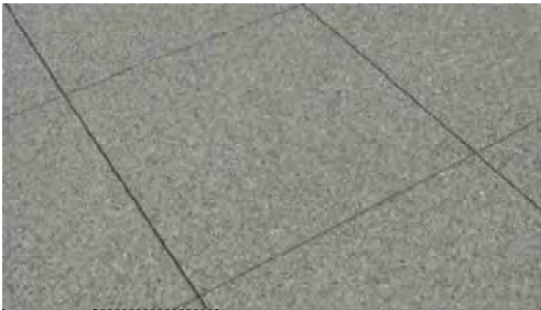
P2 CIP Concrete - Courtyard Paving
