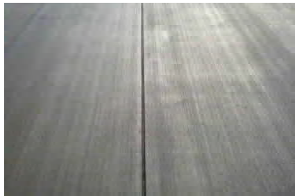
P3 CIP Concrete - Sidewalk & General
