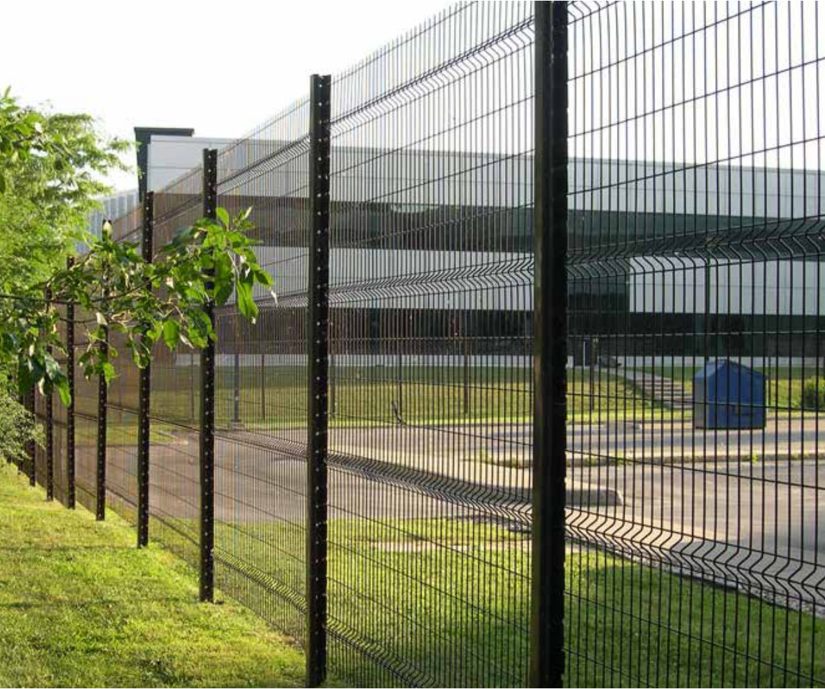
Welded Wire Security Fence, Back of Parking Garage
