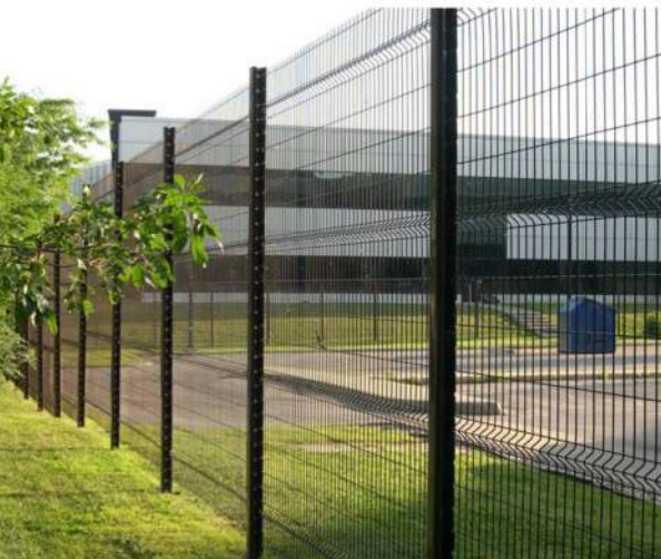
Welded Wire Security Fence, Back of Parking Garage
