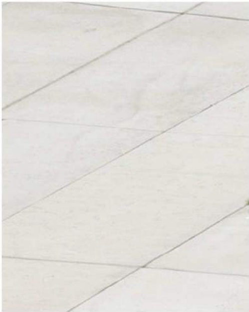
Concrete Paving with Scored Pattern
