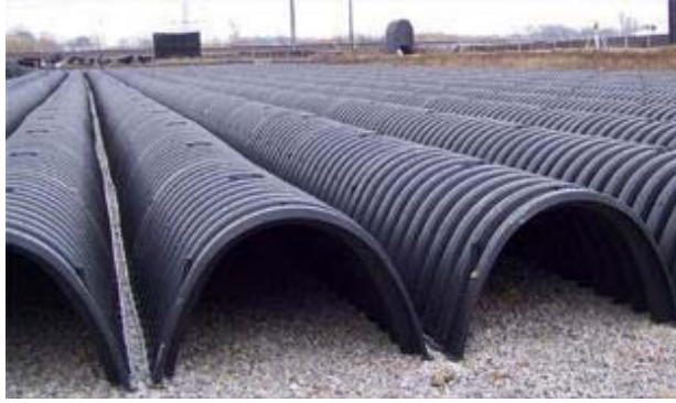
Example 1: Regional Stormwater Capture (subsurface infiltration) (Source: Conteches.com)
