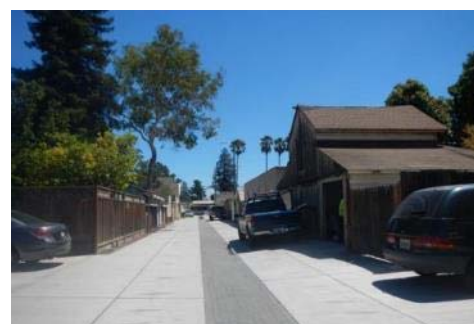
Figure 1-5. Infiltration trench covered with pervious pavement, Martha Gardens Alleys, San José (Source: City of San José)
