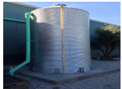
Figure 1-8. Rainwater harvesting cistern, Environmental Innovation Center, San José (Source: City of San José)
