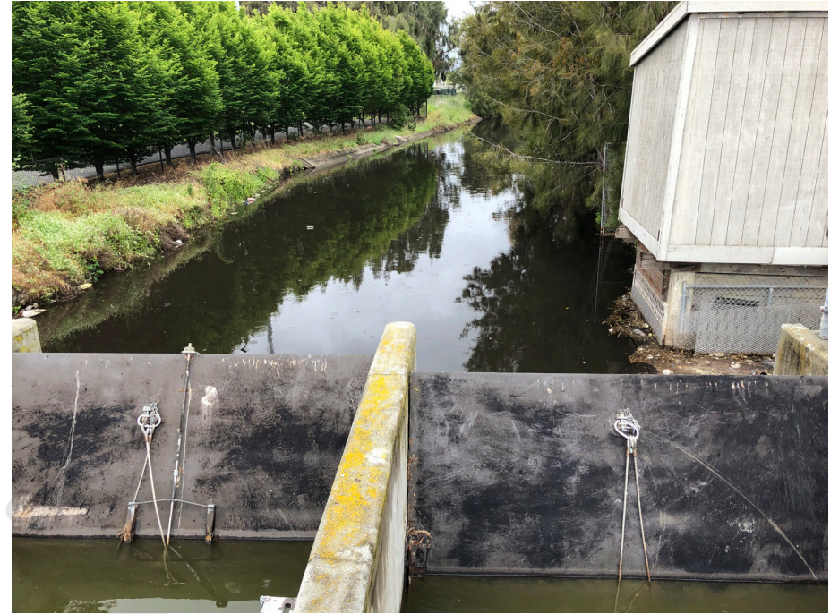
Weir Gate and Pump House at Leslie Creek Connection to Lagoon
