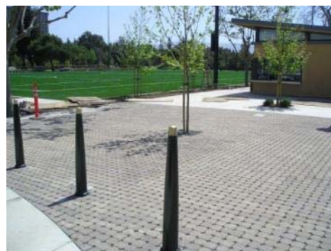
Figure 1-4. Permeable Interlocking Concrete Pavers, Mayfield Playing Fields, Palo Alto (Source: City of Palo Alto)
