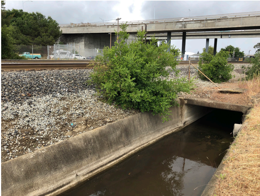
Existing Box Culvert Draining to Channel at 19th Ave and Pacific Blvd
