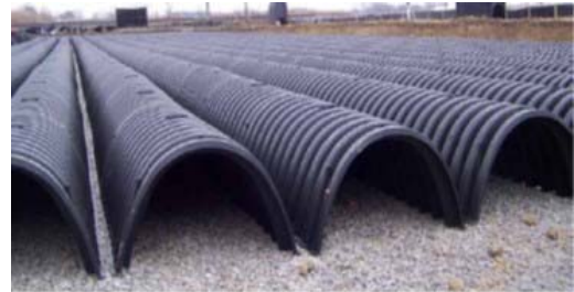
Figure 1-6. Subsurface infiltration system, generic example (Source: Conteches.com)
