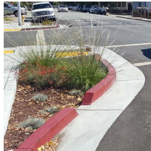
Figure 1-1. Stormwater curb extension North Central neighborhood, San Mateo (Source: City of San Mateo)
