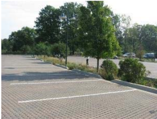
Example 2: LID (Pervious paving in a parking lot) (Source: SMCWPPP GI Design Guide)
