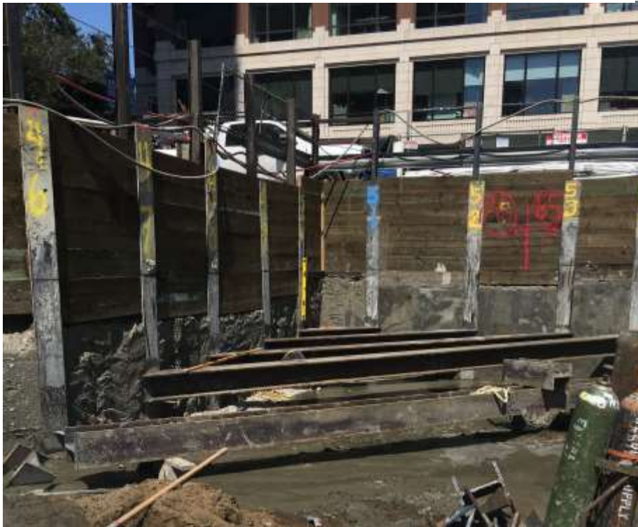
PHOTOGRAPH 6.2.2.1-3: Internal braces installed at the corner of the excavation where tiebacks cannot be installed due to utility conflicts.
