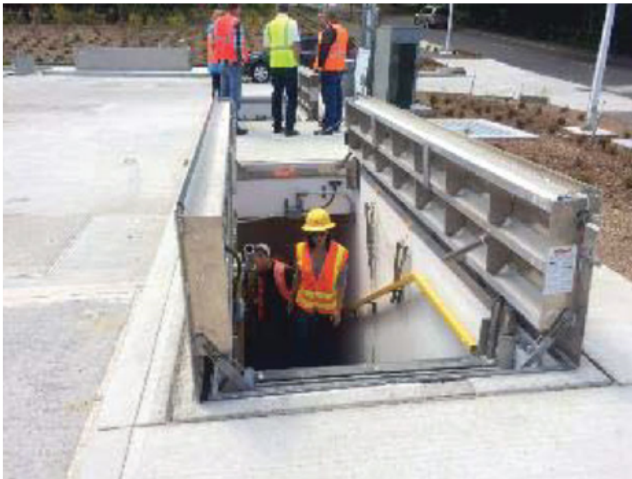
Example of ground-level air-tight vault access hatch
