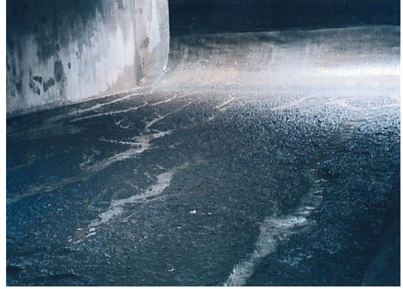
Holding structure captures solids and debris for treatment and disposal at the treatment plant
