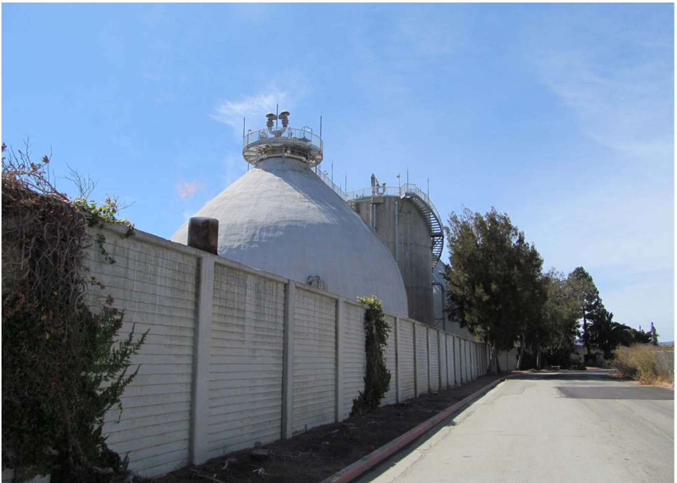
3. Detroit Drive, Existing Wall and Digesters
