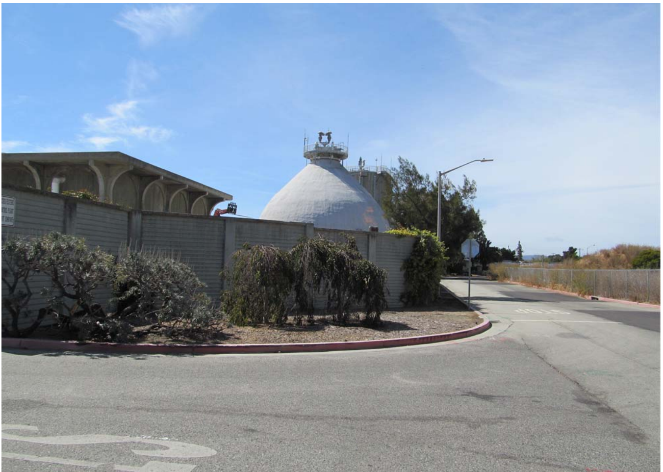
6. Detroit Drive, Looking South
