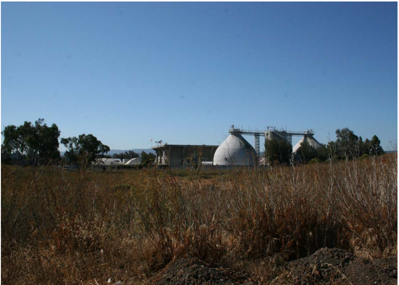
11. Project Site, Looking South
