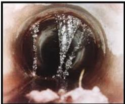
the WWTP receives flow up to 60 mgd! The difference of several million gallons is primarily caused by rainwater entering the sewer system. Cracks in pipes and separations at pipe joints allow groundwater and rainwater to enter the sewer system.
