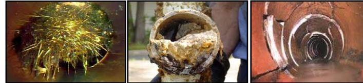
In San Mateo, blockages inside sewer pipes are most commonly caused by the intrusion of roots into sewer pipes, from the disposal of fats, oil, and grease (FOG) down drains, and pipes that are reaching the end of their useful life and have structural problems (cracks, offset joints, etc).
