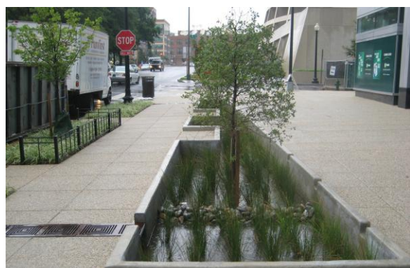
FIGURE D-18 FLOW-THROUGH PLANTER
