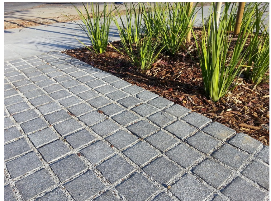
FIGURE 5-10 PERVIOUS/PERMEABLE PAVING
