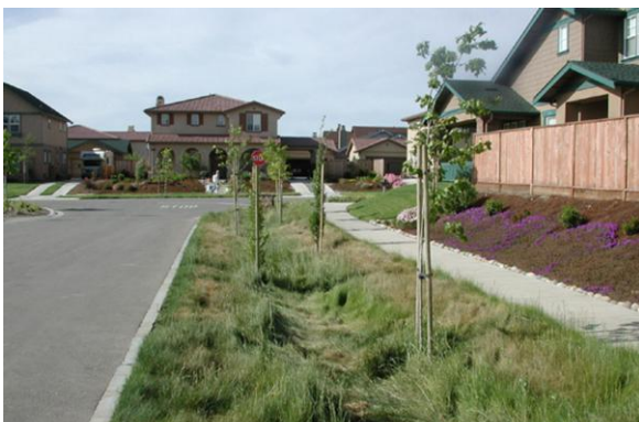
FIGURE D- 17 VEGETATED SWALE
