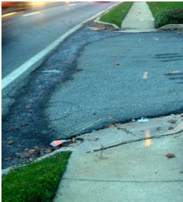
FIGURE 3-22 POOR DRIVEWAY DESIGN
