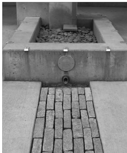
Figure IV-24 Example of permitted disconnected roof leader with splash block
