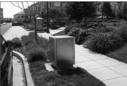
Figure III-52 Inappropriate transformer location
